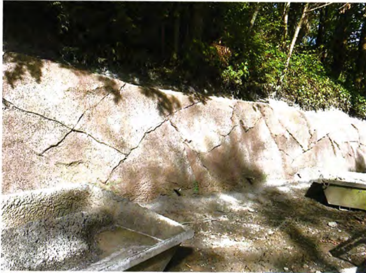
Bow Hill Road Reconstruction
