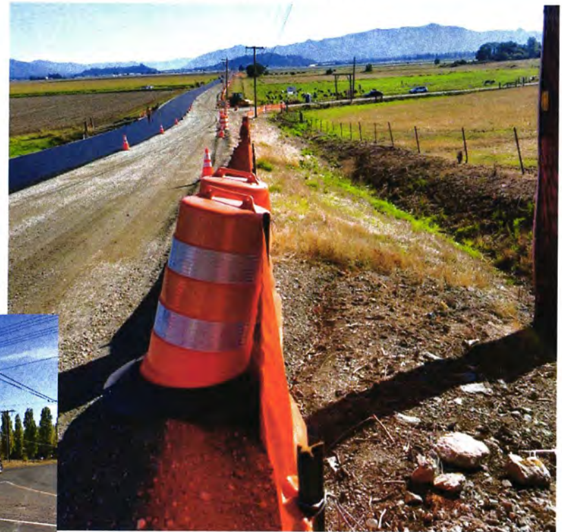
Josh Wilson Road Reconstruction
